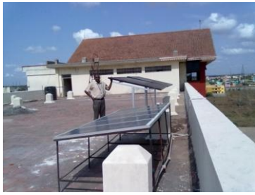
Grid-Tie Solar PV System
